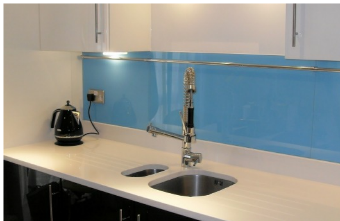
Kitchen Fitted with Glass Splashback and Showing Socket Cut-Out
