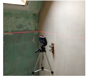
Measuring a complicated shower enclosure using Laser Technology
